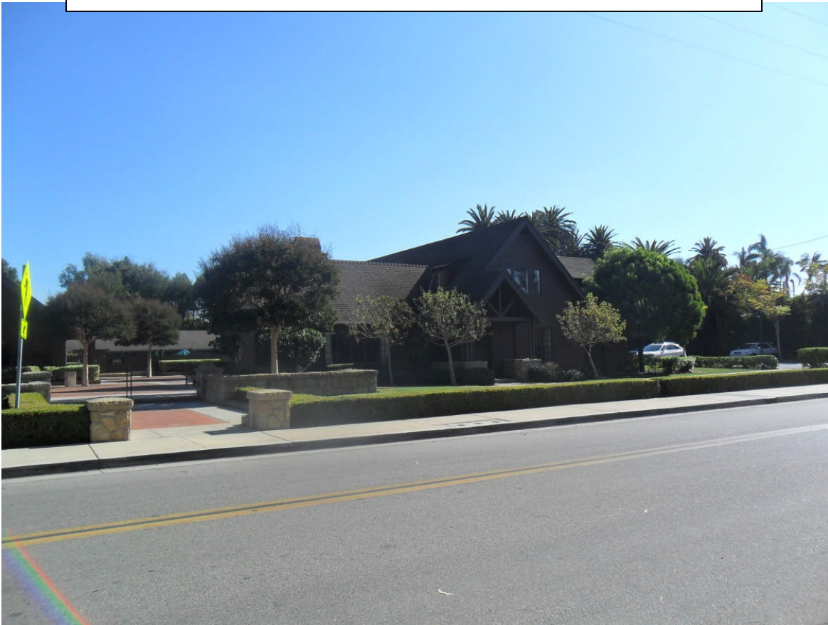
Figure 10 Centennial Hall/Parish House at All Saints By-the-Sea Church at 83 Eucalyptus Lane, Montecito Looking southeast
