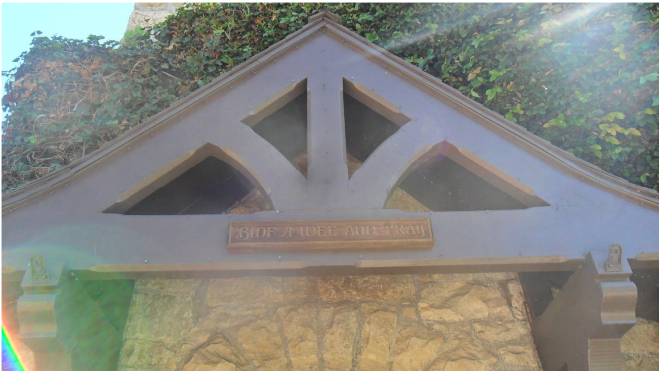
Figure 12 West elevation(primary façade), detail of porch roof Looking east
