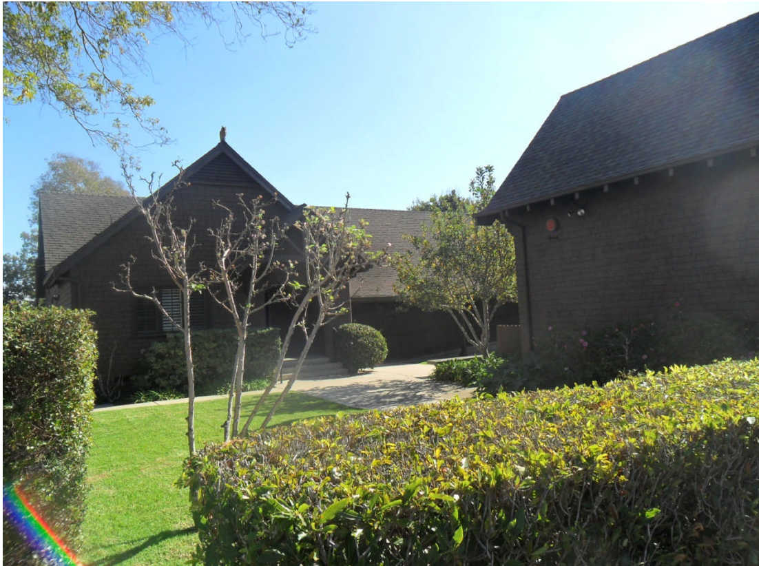
Figure 10b Parish Hall, looking east
