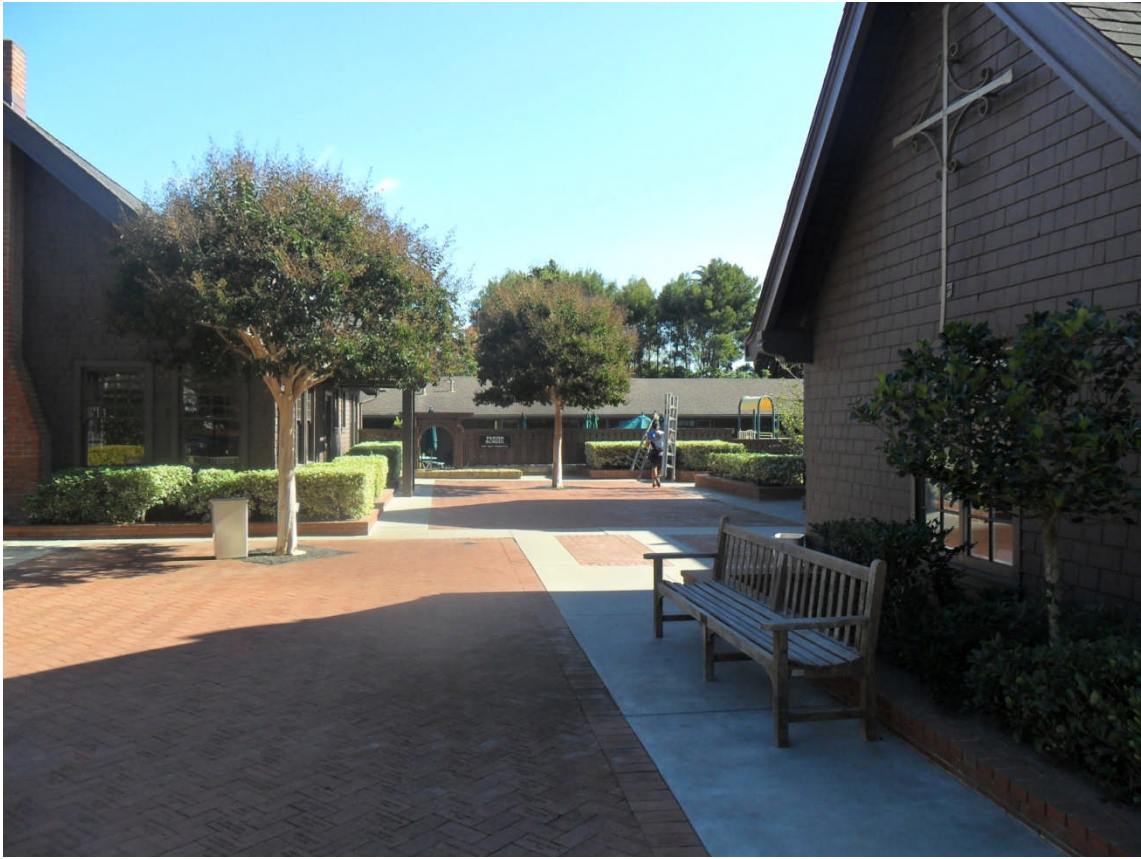
Figure 10a Classroom Building, looking east
